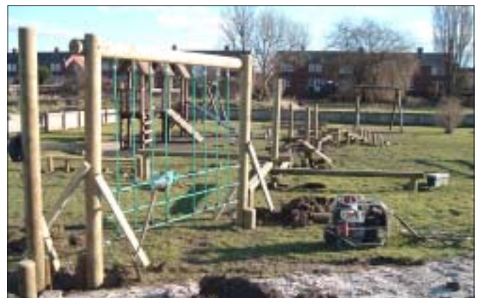
Installation of the new play equipment.
